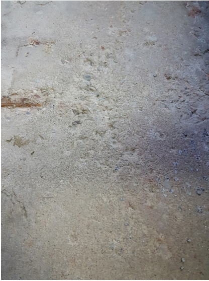
Figure 1. Shows a poor surface for reflectorless monitoring.
